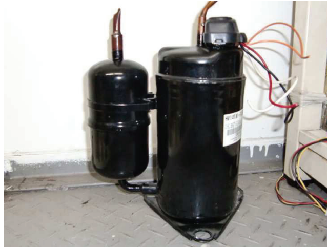
Fig. 2.7 Accumulator (left) and compressor (right)
