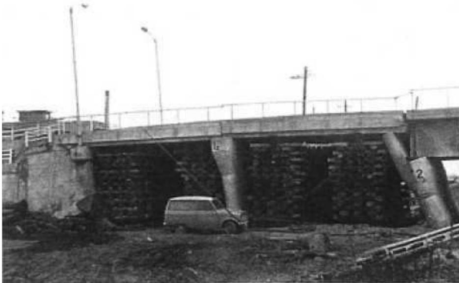
**Fig.1.3** Damages at the abutments and piers of Yachiyo Bridge (Hamada et. al, 1986)
