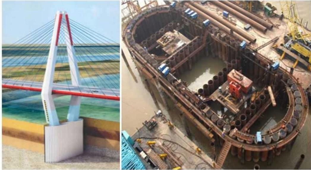
**Fig.2.2** Installment stage of SPSP foundation of Nhat Tan Bridge in Viet Nam (from <http://www.antarakoh.com.sg/contact-us.php>)
