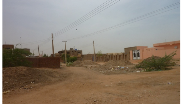
Figure 57 surface and storm water drainage challenges in Al-salama, power supply system is seen at the background
