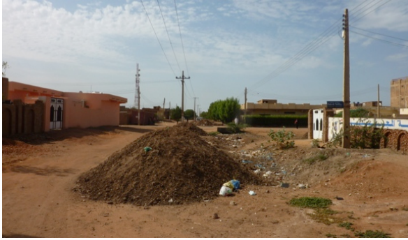
Figure 56 the f garbage collection and storm water drainage challenges observed in Al-salama
