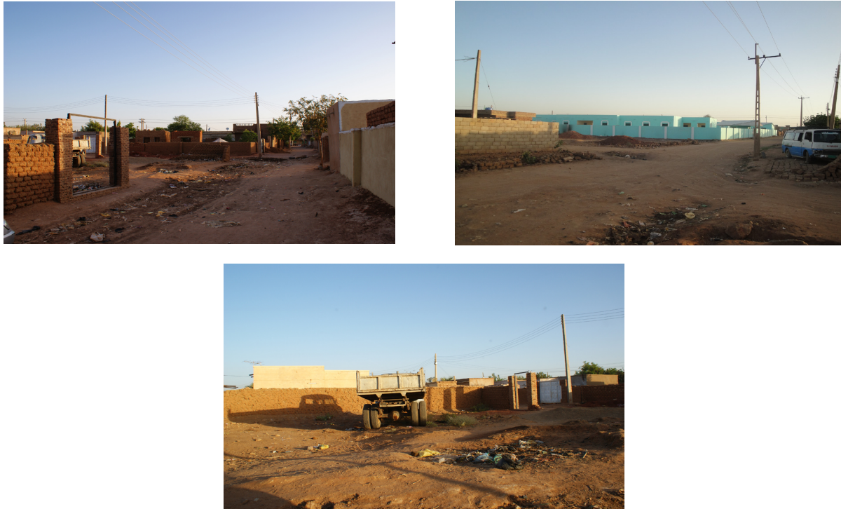
Figure 36 surface drainage and solid waste challenges in Al-shigla neighbourhood
