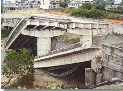
Figure 1.3 The bridge collapsed during the 1999 Chi-Chi earthquake. (Source: http://whatiscivilengineering.csce.ca/structural_earthquakes.htm )
