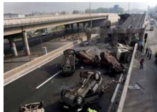
Figure 1.5 A bridge collapsed in Santiago during the 2010 Chile earthquake. (Source: AFP, REUTERS).
