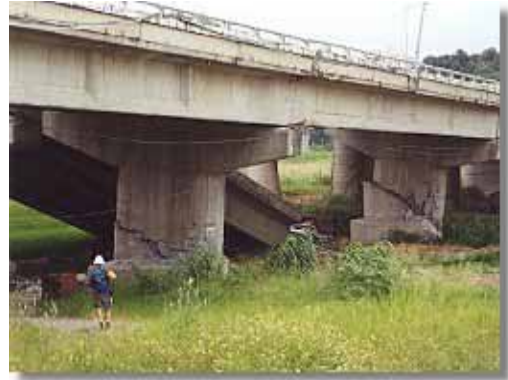
Figure 1.3 The bridge collapsed during the 1999 Chi-Chi earthquake. (Source: http://whatiscivilengineering.csce.ca/structural_earthquakes.htm )
