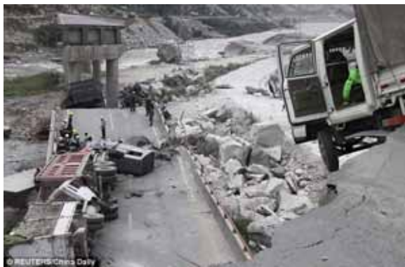
Figure 1.4 A bridge collapsed in Santiago during the 2008 Sichuan earthquake. (Source: http://www.dailymail.co.uk ).
