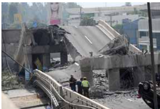
Figure 1.5 A bridge collapsed in Santiago during the 2010 Chile earthquake. (Source: AFP, REUTERS).
