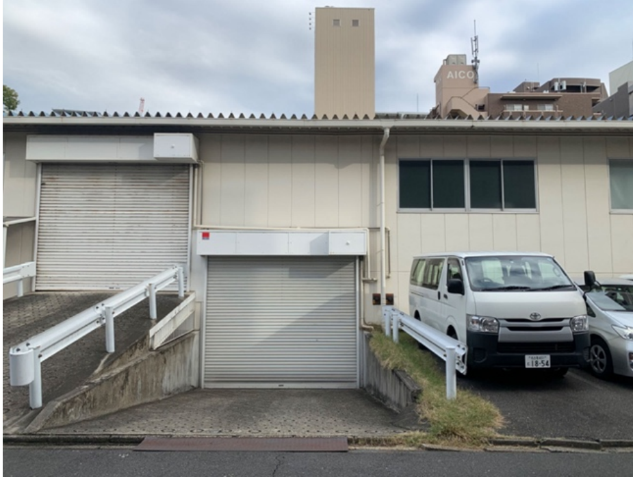
Fig. 4-37 Office building in Shikemichi area without historical elements (Photo in 2022.11, author)
