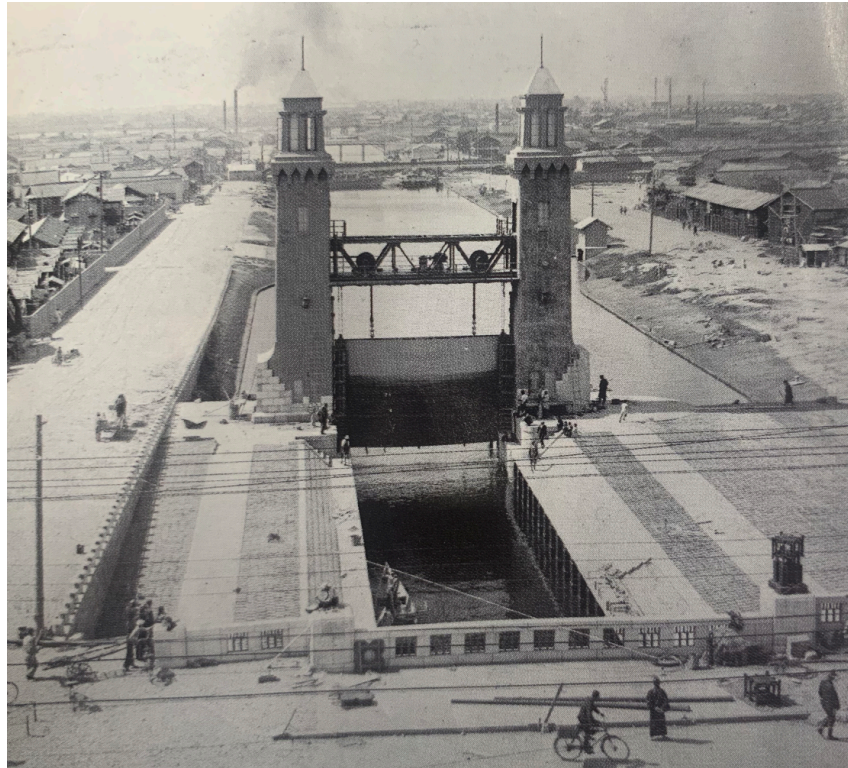
Fig. 1-5 Matsushige sluice gate nearing completion in 1932 (Source: Nagoya City Archives)
