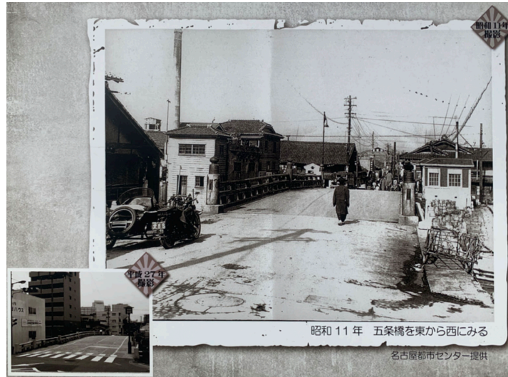
Fig. 1-7 A photo of the Gojo bridge taken in 1936 (Source: Nagoya Urban Institute)
