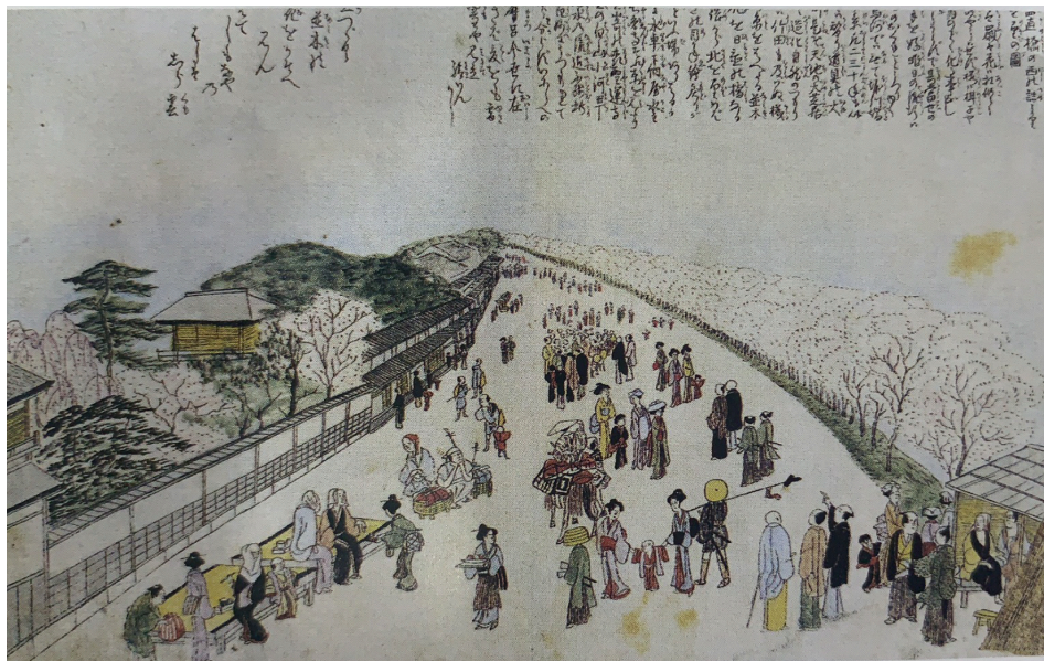
Fig. 1-14 View from the north-west of the Hioki Bridge (Source: 高力種信, 2006 36 )
