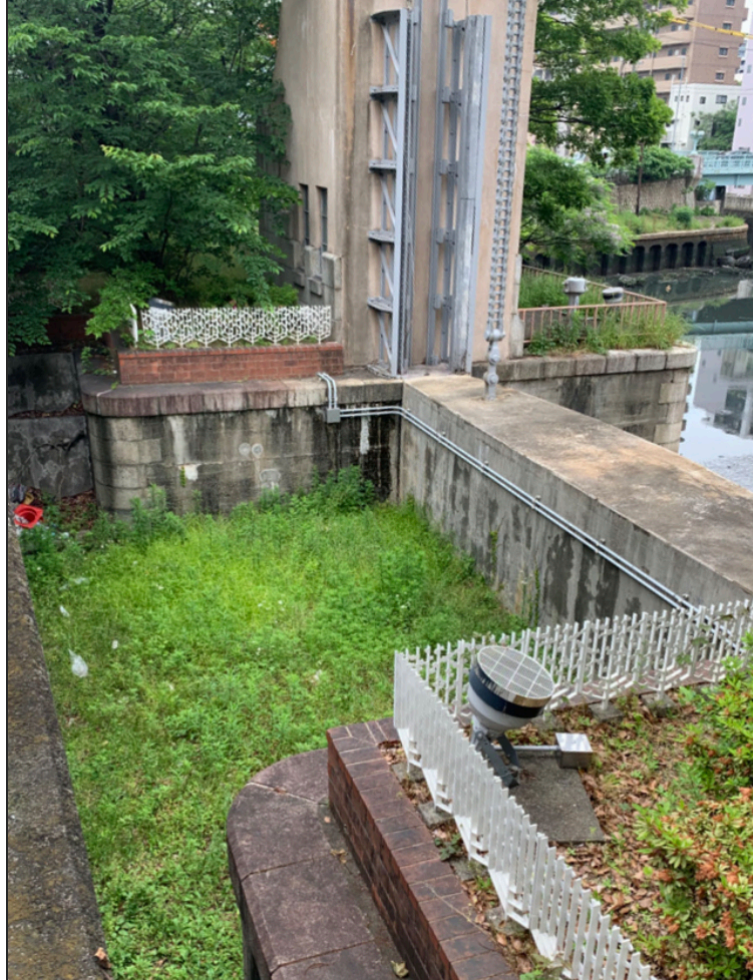
Fig. 1-16 The closure of the Matsushige sluice gate (by author, 2022)
