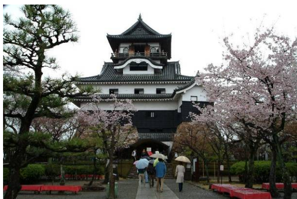
(a) Exterior view.
