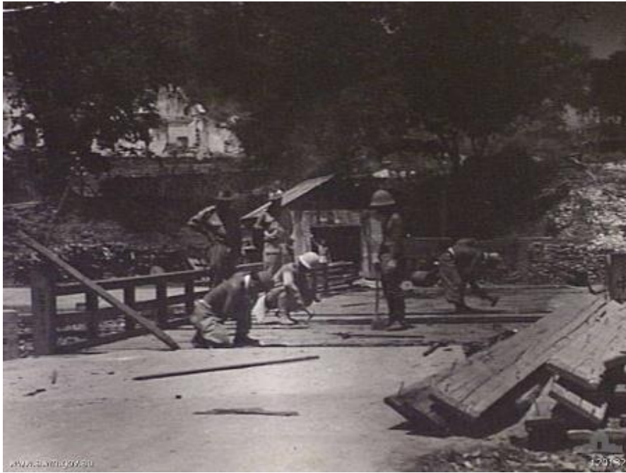
Figure 50. Japanese POWs repairing a bridge.
