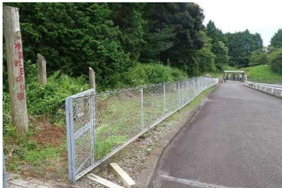
1) Fence, Asphalt, Slope
