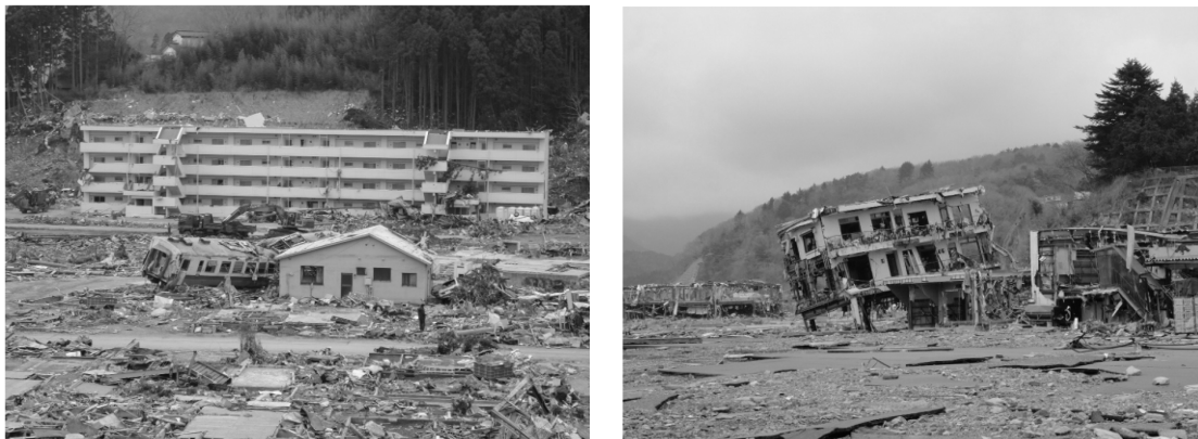
Figure 1-1. View after tsunami (courtesy of Junji Katsura).
