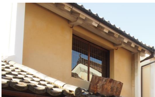
Fig.3.16 Roof eaves with visible deketa , 2015.
