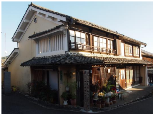
Fig.3.18 Zashiki-type house, 2015. The second-floor windows, with glass fixtures and dobukuro box, but the study in 1978 did not state clearly whether they were considered traditional or not.
