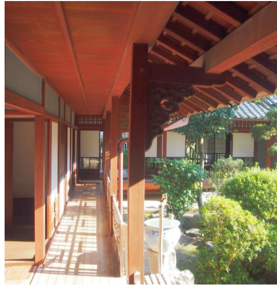
Fig.3.40 Mochiokuri-deketa-pillar structure in Kamihaga house, 2015.
