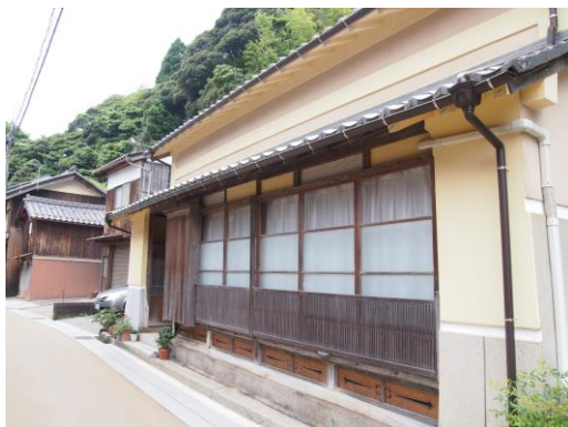
Fig.4.48 Ine, 2016. A small lattice convertible to bench for trading.
