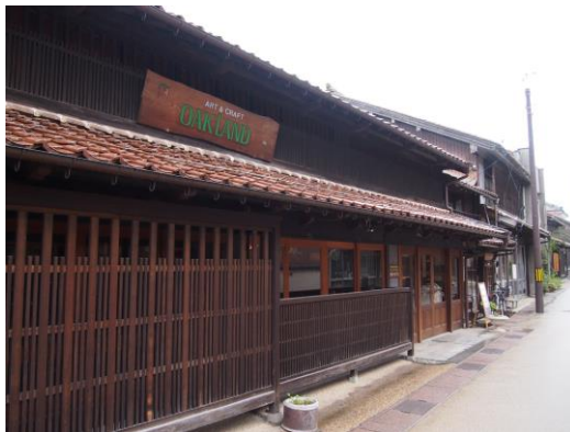
Fig.3.57 Kurayoshi, 2015. Different lattices for different spaces in the mise.
