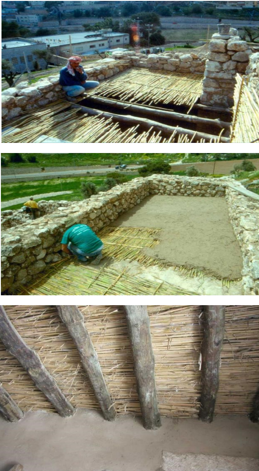
Figure 3-16: Example of the roof materials and construction methods (NA, 2017)
