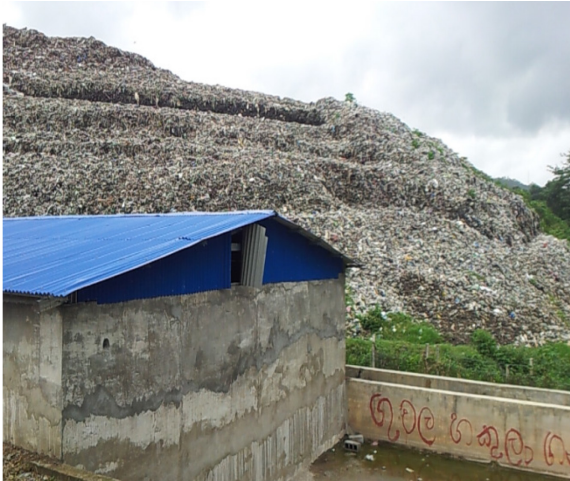
KANDY open dumping site
