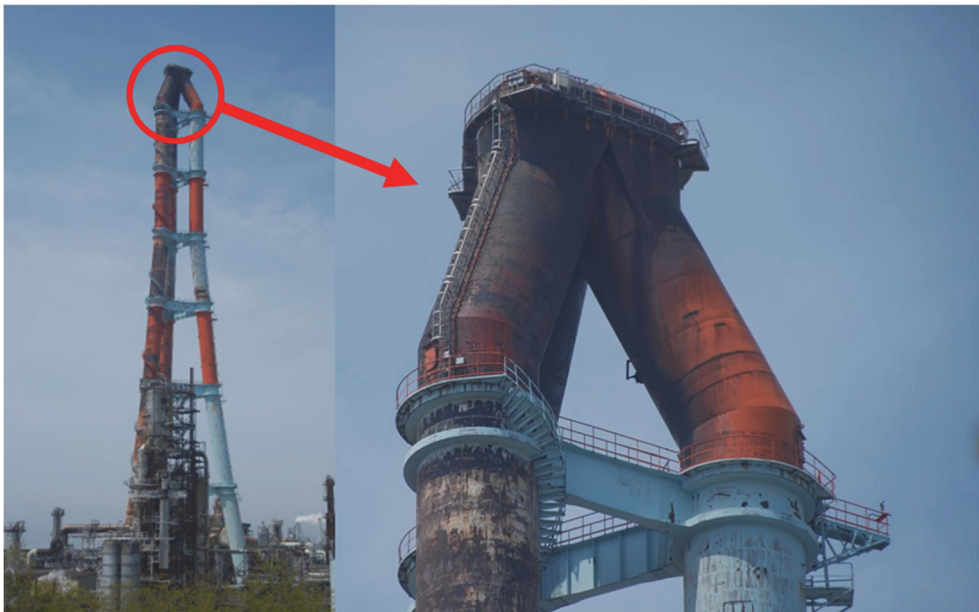
Fig. 1.6 High-rise chimney and ladders on it [15].
