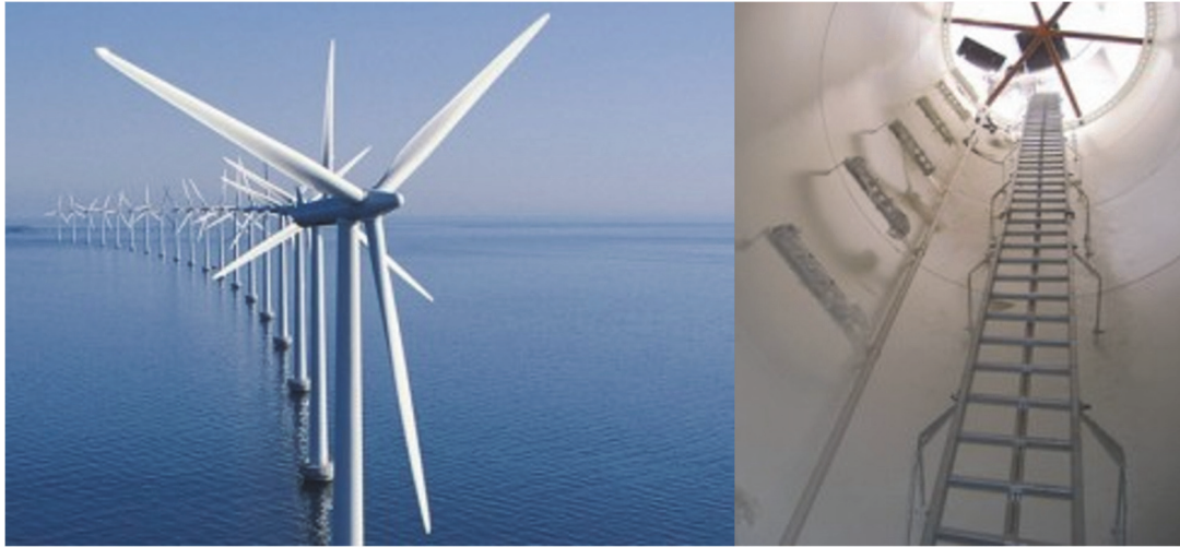
Fig. 1.5 Off-shore wind turbine and the ladder inside ([13], [14]).
