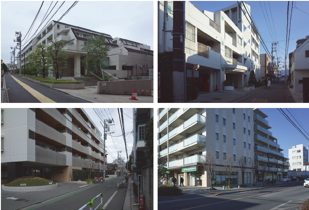
Figure 6-52 Building setback in case No. 01, 03, 07, 08 (Photos by author, 2017)
