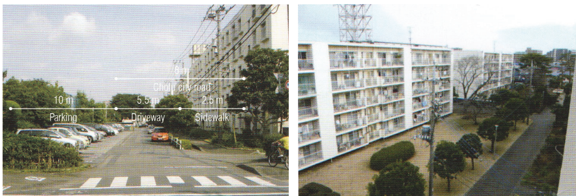
Figure 6-37 Chofu Fujimi Housing before reconstruction (Left: street to the north and parking with dimensions; Right: pedestrian in the middle of the plot; Source: Asahi Kasei)
