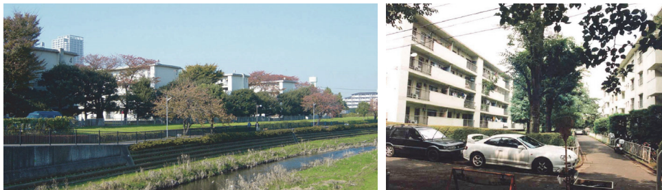
Figure 6-17 Condition of Kokuryo Housing before reconstruction (Source: Asahi Kasei)
