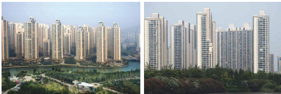
Figure 1-3 High-density residential area in redevelopment project of Zhongyuan Liangwancheng in Shanghai (Photos by author, 2010)
