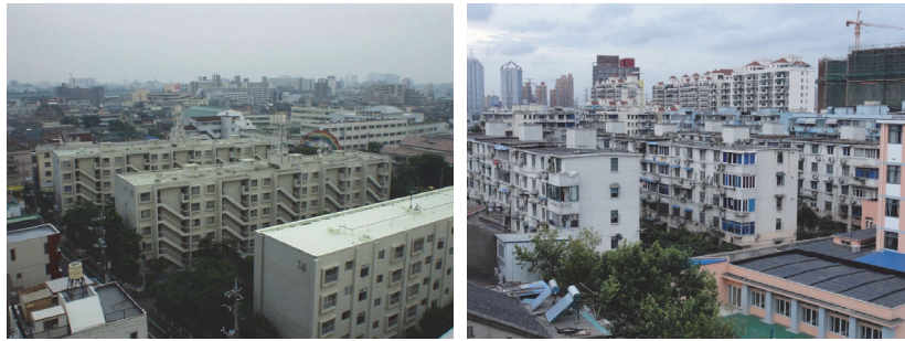
Figure 4-10 Haginaka Condominium Complex in Tokyo, completed in 1968, before reconstruction (left, source: マンション再生協議会) and Lantian New Village in Shanghai, completed in 1983 (right, photo by author, 2015)
