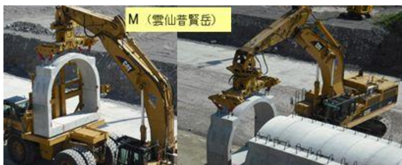
Fig. 1.14 Box culvert [1.3]
