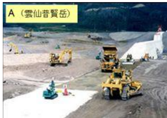
Fig. 1.9 Compacted concrete [1.3]
