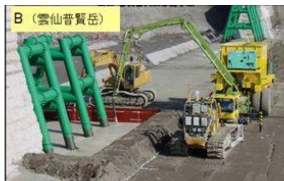
Fig. 1.10 Steel slit [1.3]
