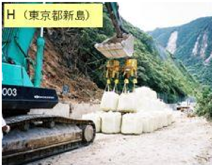
Fig. 1.13 Placing sandbags [1.3]
