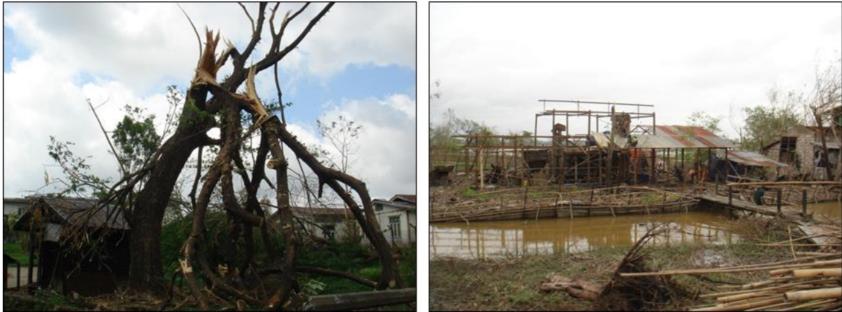
Figure 2.4 Debris due to cyclone Nargis found at Letkegon, near Yangon (Shibayama et al. 2009)
