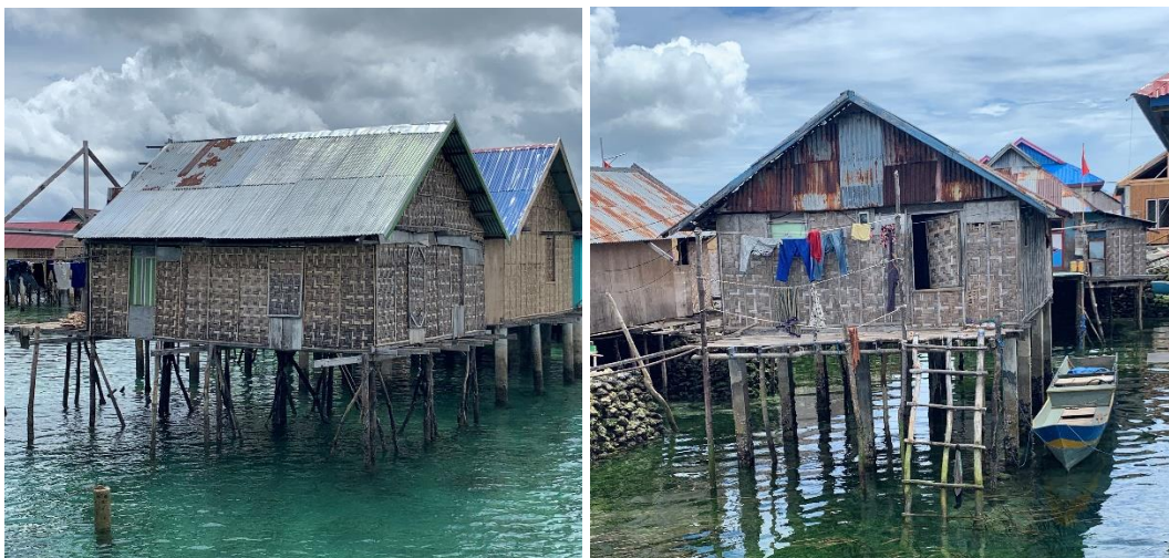
Figure 38 Wooden houses on wooden stilts (left) and concrete stilts (right) (source: field study)
