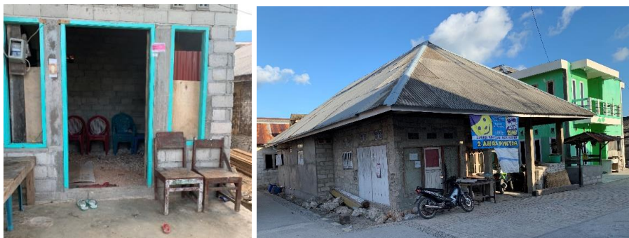
Figure 39 House made from concrete bricks
