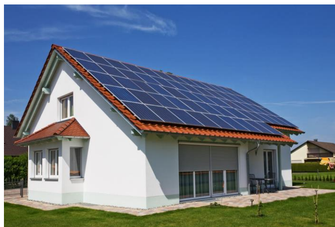
Fig. 2.2 Example of PV system used on roof.
